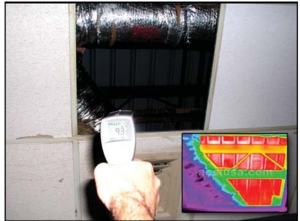
IHOP (Below Uncoated Roof)
